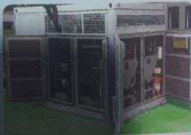
2 x 40kVA EMI/EMC proof compact DG Set with 16kVA UPS for Aakash NG
